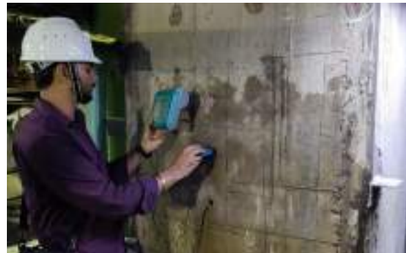
Half Cell Potential Measured Column
