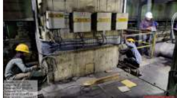
UPV Test on TG Column
