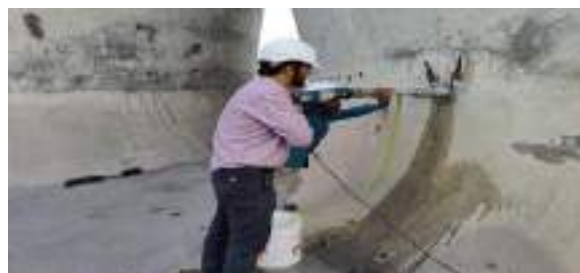
Core Extraction from the RCC SHELL
