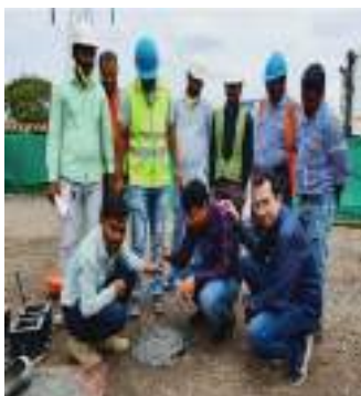
Measurement of slump of geopolymer concrete mix being taken at site
