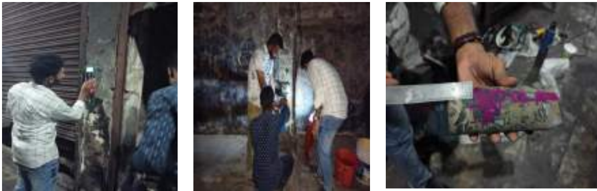
SAR (NDT) Testing of Building at Puri, Odisha
