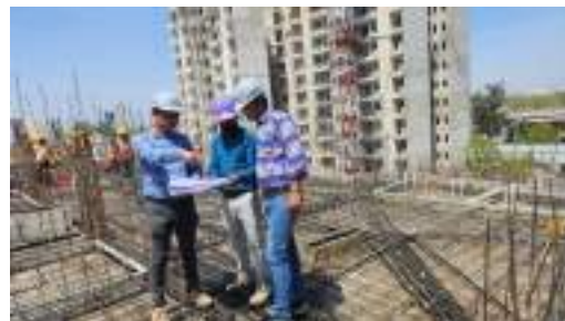
Checking of reinforcement at Residential Accommodation at Kasturba Nagar, Delhi
