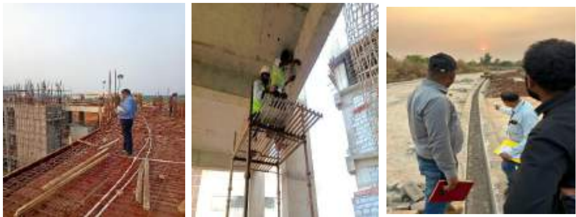
TPQA Site Inspection Project at NBCC IIT Bhubaneswar Project Site
