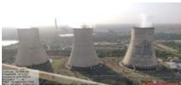
Project site of Condition Assessment of RCC NDCT Cooling Tower
