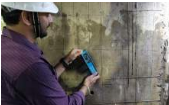
Electrical Resistivity Measured on TG Column
