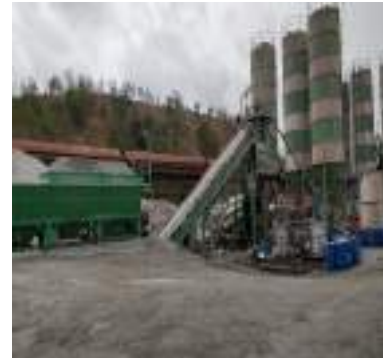
Batching plant setup for the production of geopolymer concrete mix
