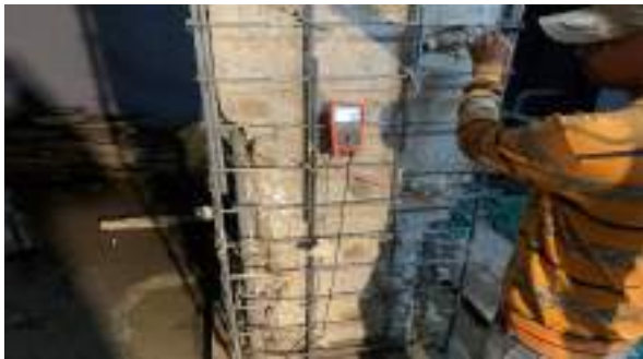
Continuity testing being done after installation of Zinc anodes at site
