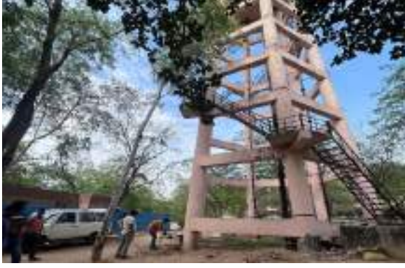
Non-Destructive Test Evaluation Technique for 4 Nos Column of Overhead Water Tank at RAF Vastral, Ahmedabad-Reg- Central Public Works Department- Ahmedabad
