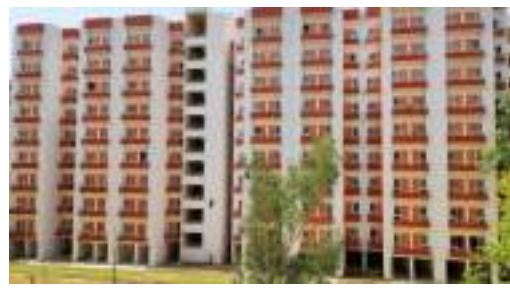
General Pool Residential Accommodation at Thyagraj Nagar, Delhi
