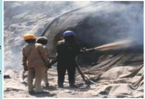
Shotcreting of NCB-Quick set formulation inside tunnel at a dam site
