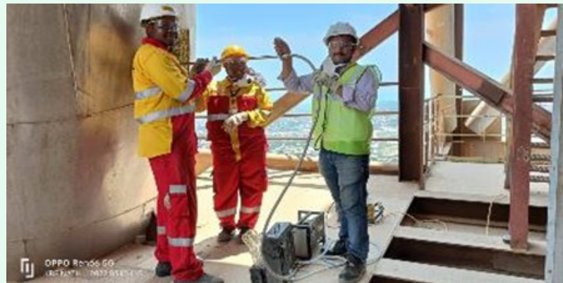
Measurement of moisture in flue gases
